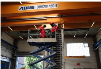
After we attached the lower 6 hoses, Halil took me up on a scissor lift platform to the top of the 6 meter tall spiral conveyor.
