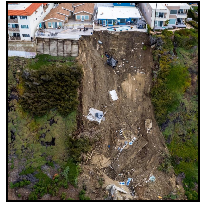
Figure 1: A March 2023 Landslide in San Clemente, California [1]
